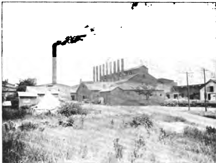
A. PLANT OF THE PEERLESS PORTLAND CEMENT COMPANY, UNION CITY, MICHIGAN.
